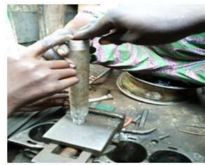
(c) Welding of the gas inlet pipe to the chamber of the mixer device
