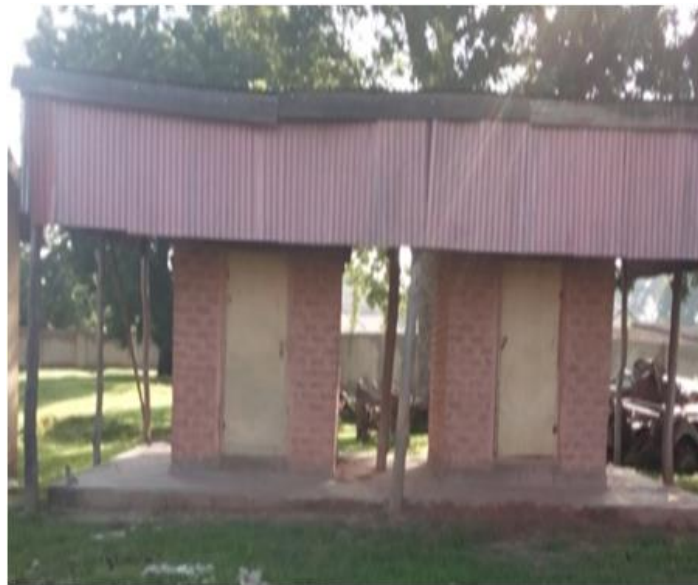
Fig. 2 Pictorial view of the constructed rooms
