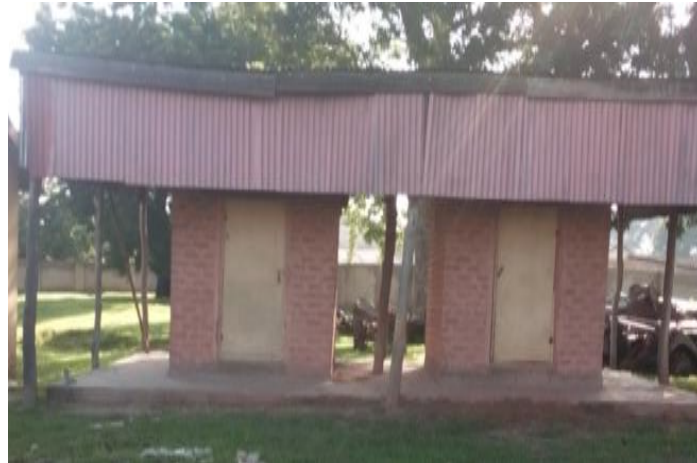
Plate1 Pictorial view of the constructed cool rooms indicating the applied natural cooling
