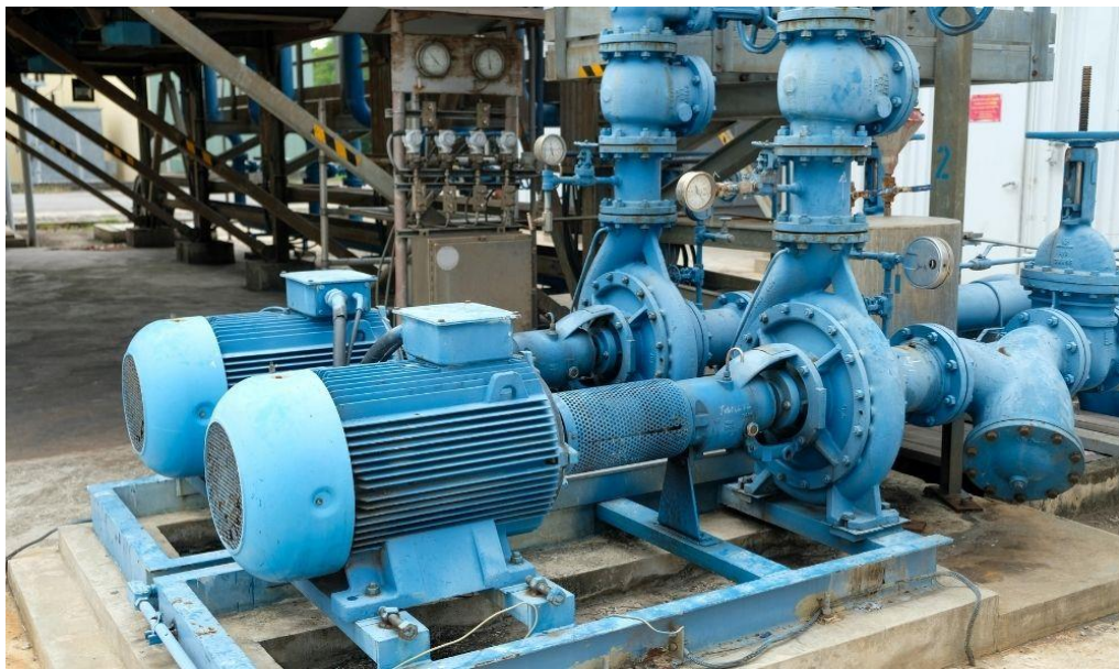
Fig. 1 Installed Centrifugal pumps (in series) in the wastewater treatment plant (WRPC, 2025)
